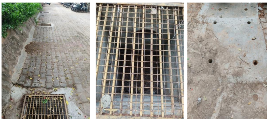
Figure 4-10: Percolation pits for rain water harvesting
