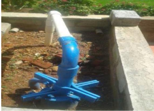
Figure 4-12: Point recharge for a Bore well
