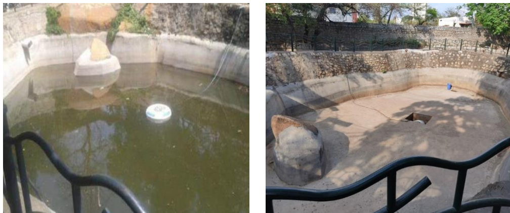
Figure 4-7: Rain water harvesting pond
